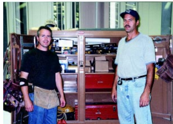
The Reference renovation underway
